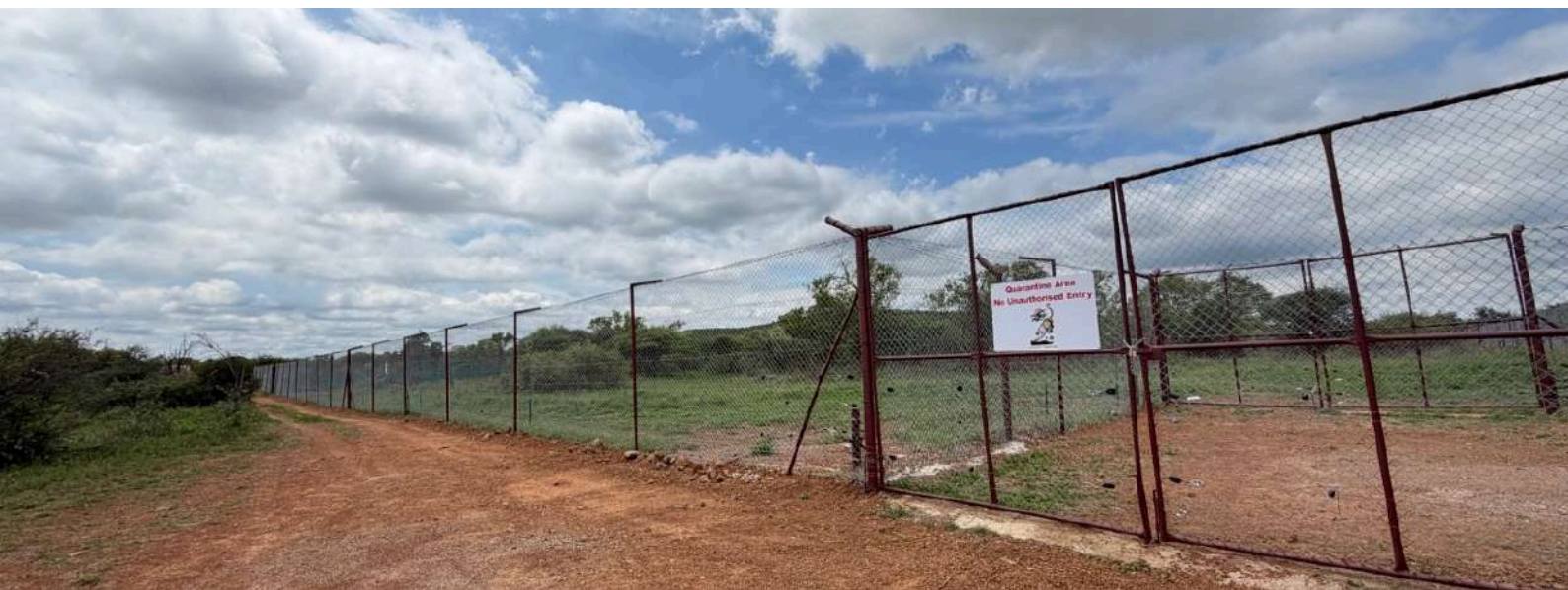
Upgraded Quarantine Facility at Mokolodi Nature Reserve, Gaborone
